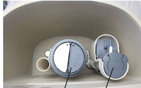
Flush Valve Fill Valve
