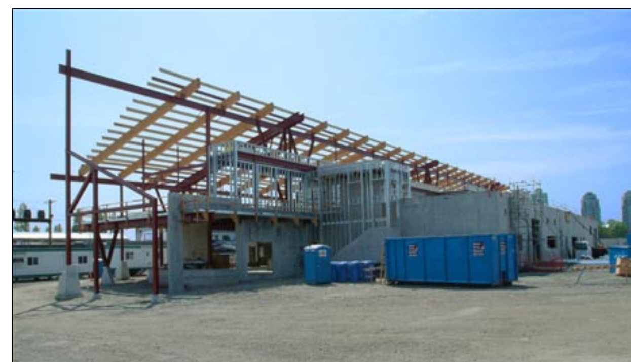
ADMINISTRATION BUILDING UNDER CONSTRUCTION
