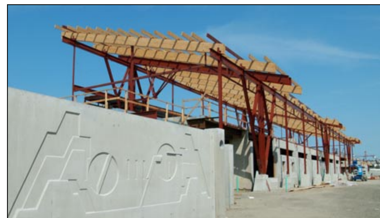
ADMINISTRATION BUILDING UNDER CONSTRUCTION
